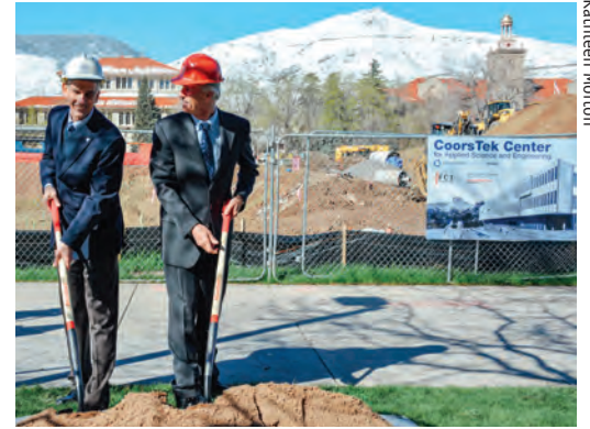
CoorsTek CEO John Coors and Mines President Paul Johnson break ground on the new CoorsTek Center for Applied Science and Engineering.
