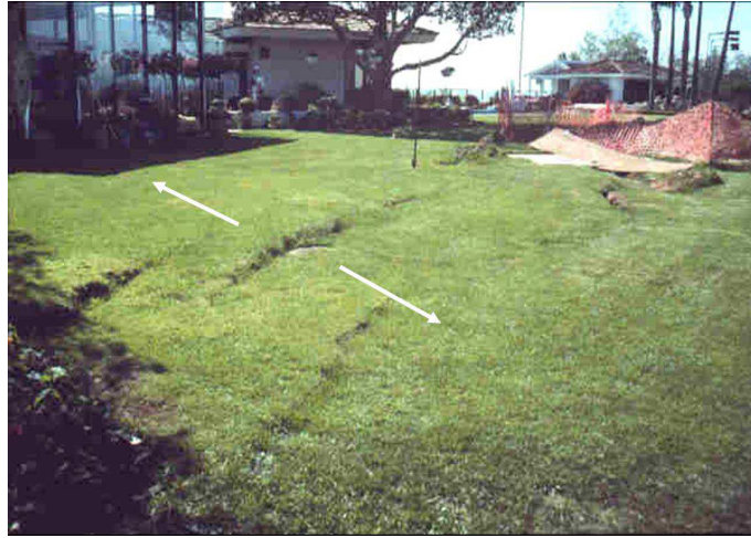
Figure 1.4. Photograph taken after the Northridge, CA earthquake in 1994 showing extensional cracks caused by the dynamic stress of the earthquake (from Randall Jibson, U.S. Geological Survey)
