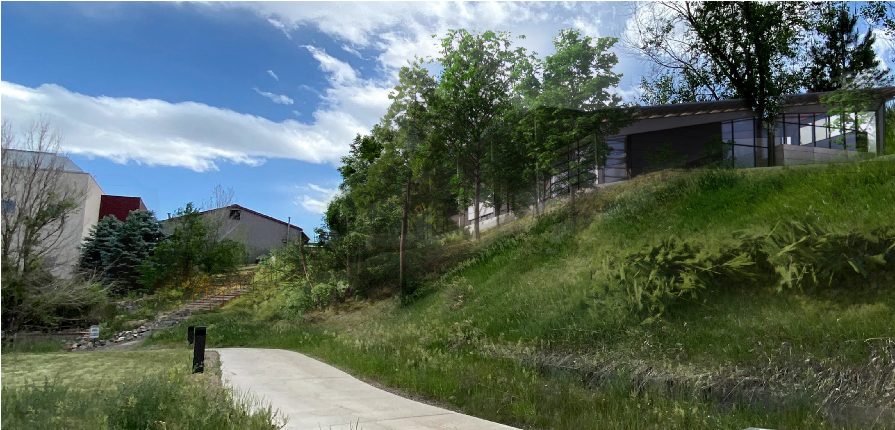
VIEW OF SITE FROM NORTH WITH BUILDING
