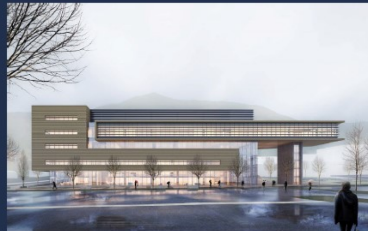
Minerals and Energy Resources Building
