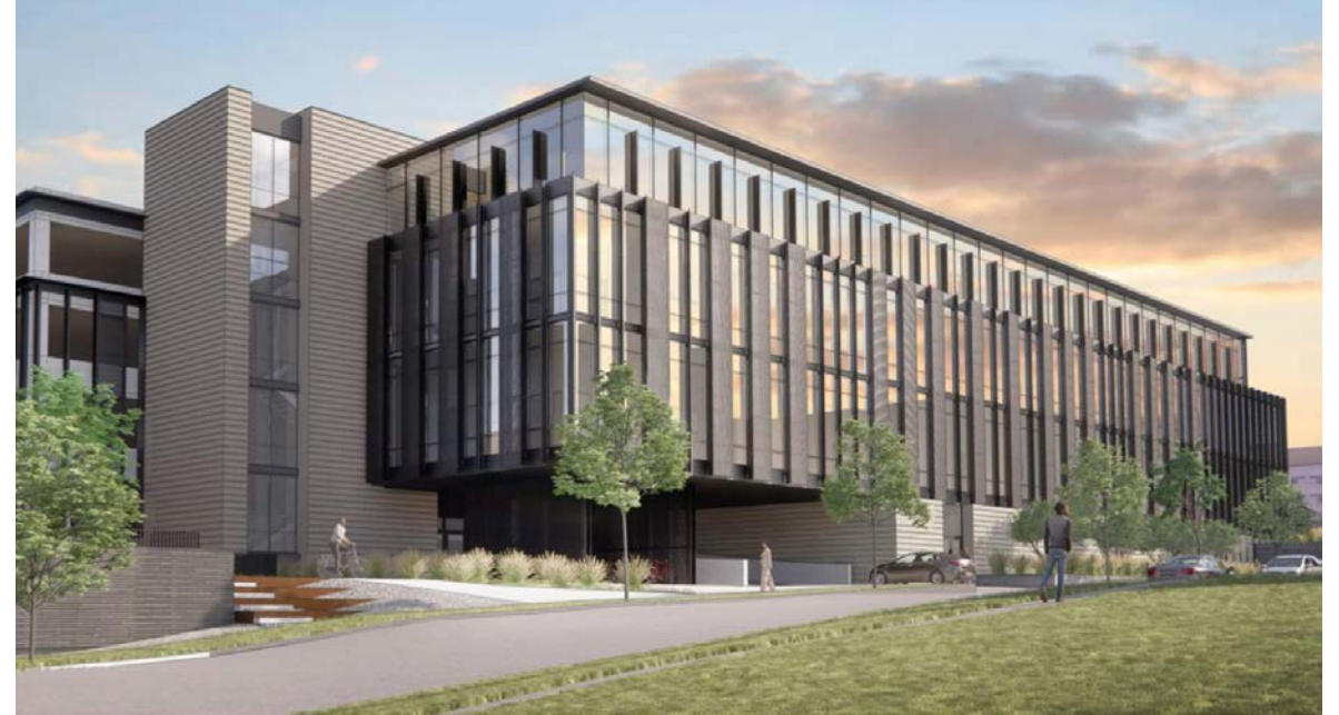
Looking Southwest from 17 th & Washington
