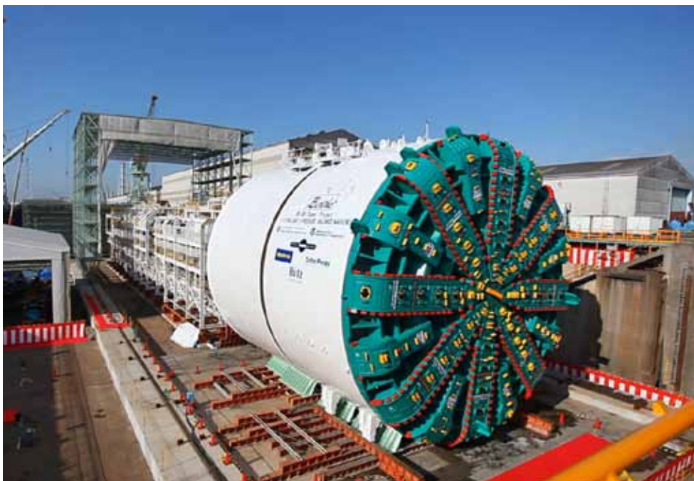
The SR 99 tunneling machine in Japan.
